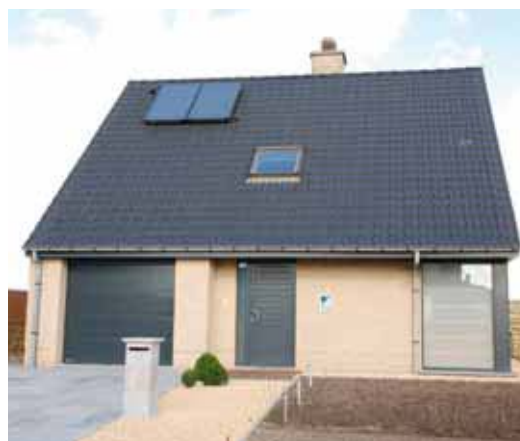
➤ The Daikin Energy Saving House real-life environment offers perfect test conditions for Daikin's advanced heat pump technology.
