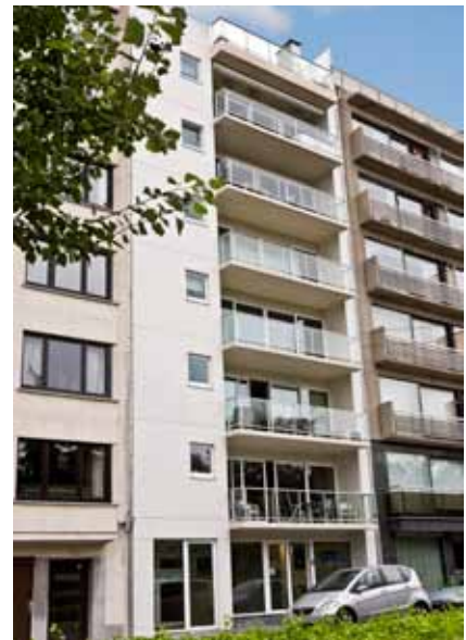
➤ The Daikin Apartment in Ostend, Belgium
